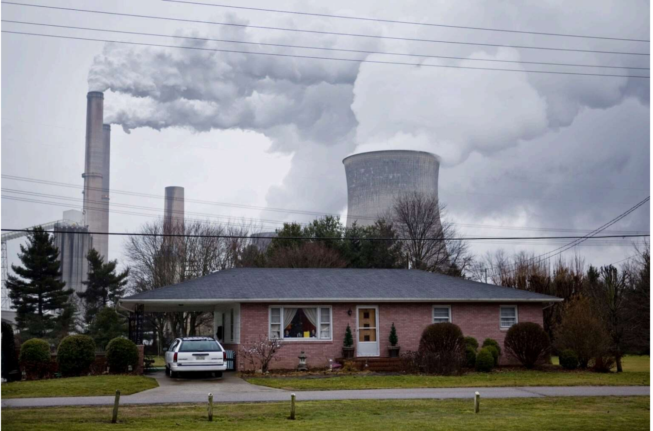
The stacks from the Gavin power plant behind a nearby home in Cheshire, Ohio. Image: Benjamin Lowy/Getty Images
